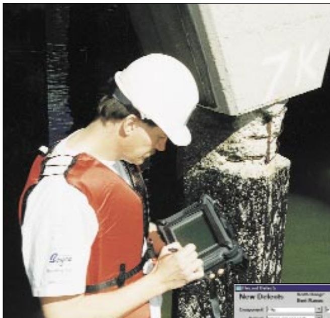
The inspector inputs data for each specific defect, allowing systematic development of an estimate using the AIRIS program.
