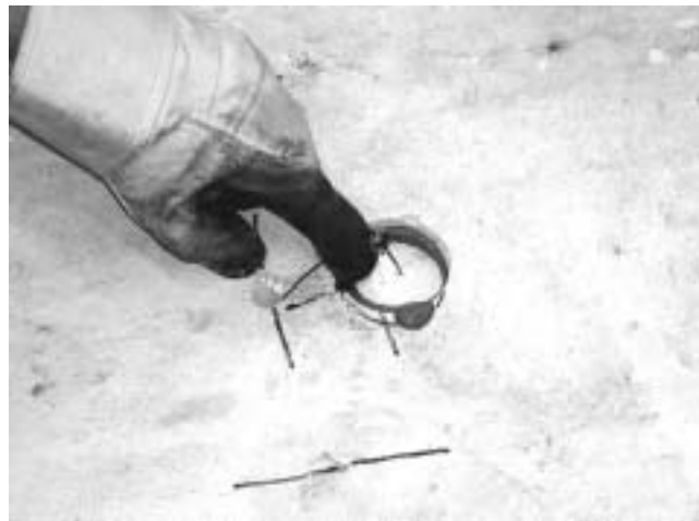
Fig. 13—Anode placed in hole with patching material.
