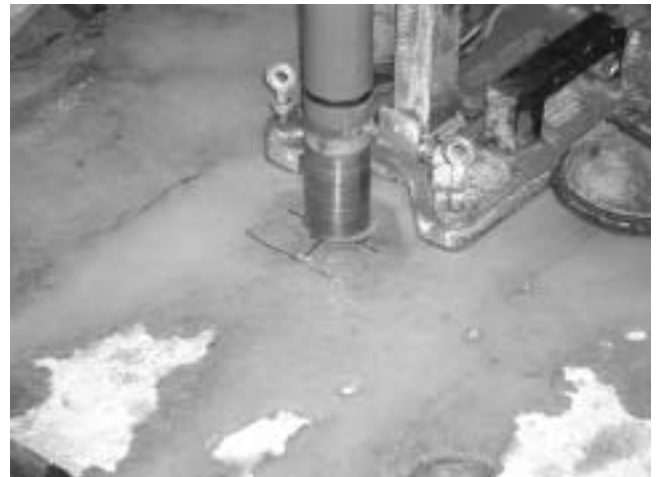
Fig. 10—Coring hole for anode.
