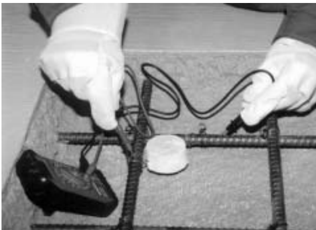
Fig. 8—Confirming connection to reinforcing steel.
