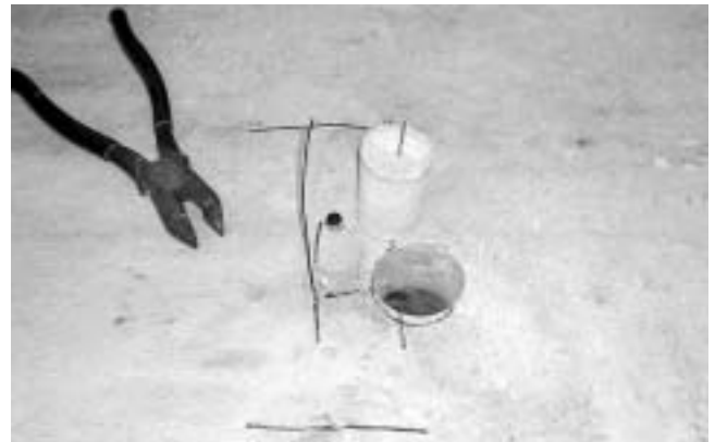
Fig. 11—Secondary hole with reinforcing steel connection.
