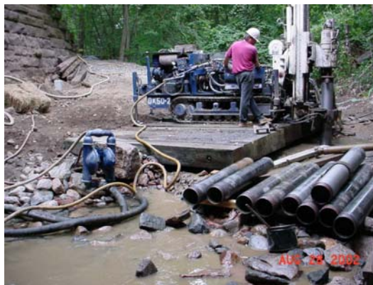
1. Sacrificial Test Pile
