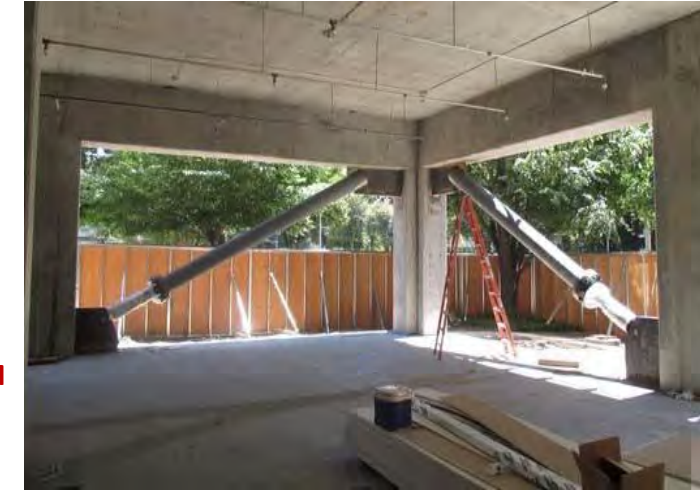
Flood Viscous Dampers
