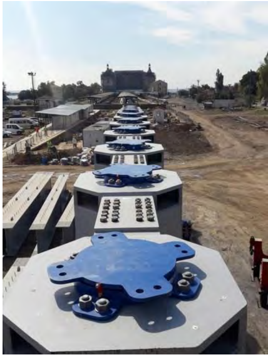
Friction Pendulum Bearings
