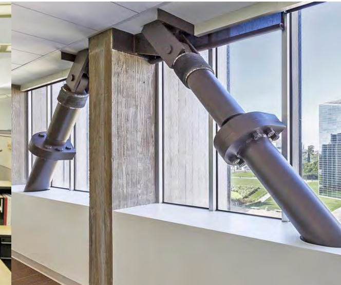
Flood Viscous Dampers
