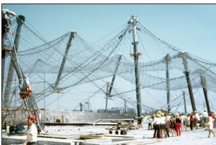
Fig. 4: Tentlike roofs for the Olympic Games in Munich (1968–1971)
